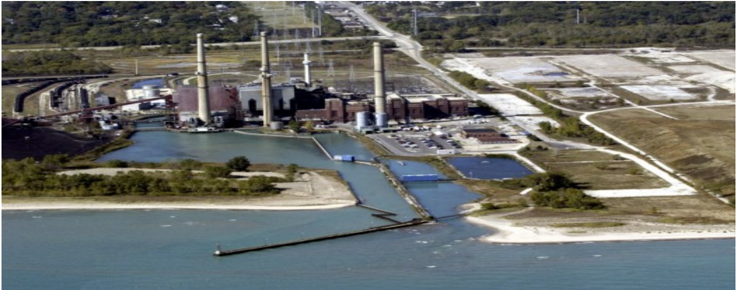
Aerial photo of Midwest generation plant (left) with Johns-Manville site (right).
