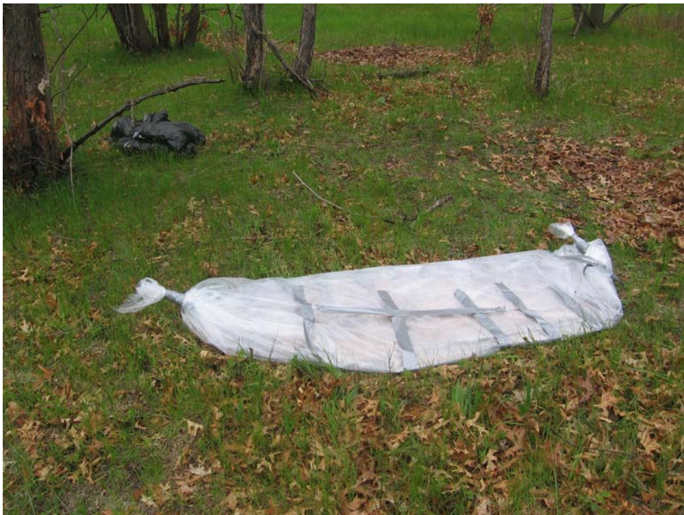
Figure 4 - Wrapped, Unlabeled, and Unsecured Waste in Kellogg Creek Area Regulated Asbestos is wrapped, unlabelled, in a dry condition, then left unsecured overnight.
