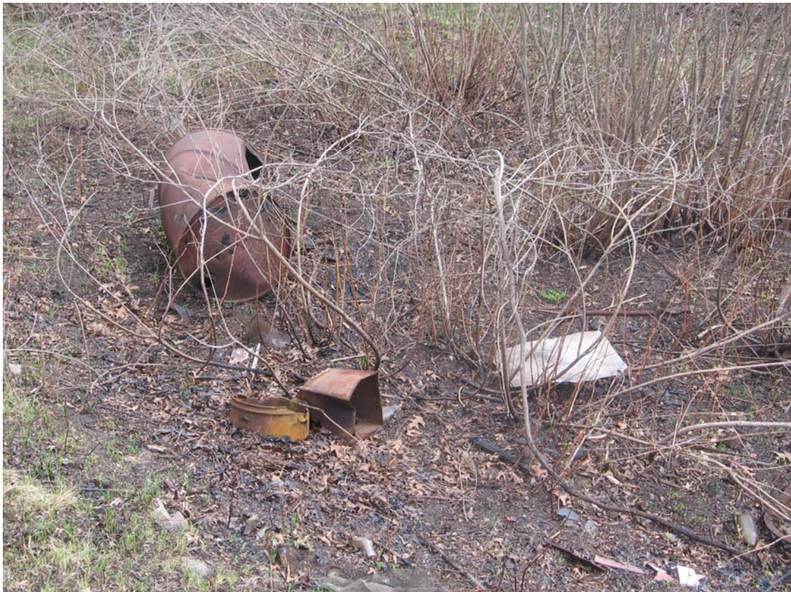
Figure 4 – Asbestos debris (white material on right side of photo) is mixed with dangerous demolition debris which creates a hazardous environment in unrestricted public areas at Illinois Beach State Park.
